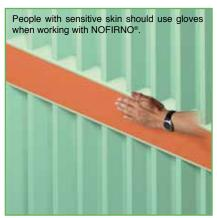
7) The surface can be smoothed by hand. Wet the hands thoroughly with soap and water to avoid the NOFIRNO® sticking to the hands. A very neat surface is the result. Prevent soap water to be applied on the sealant surface on which the next sealant will be applied.
