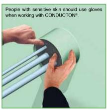
9) Firmly press down the mass once more by hand. This is extremely important to ensure effective conductivity. Then apply the CONDUCTON® flexible rubber at the other side of the penetration in a similar way.
