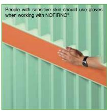
7) The surface can be smoothed by hand. Wet the hands thoroughly with soap and water to avoid the NOFIRNO® sticking to the hands. A very neat surface is the result. Prevent soap water to be applied on the sealant surface on which the next sealant will be applied.
