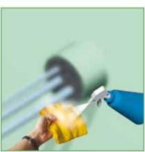
11) To smooth the surface of the FIWA® sealant layer, a cloth is sprayed with water. This prevents the sealant from sticking to the cloth. Note: do not use soap water!
