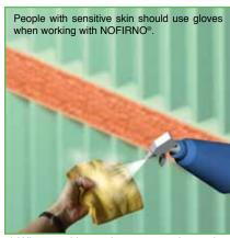
5) When working on larger gaps, the sealant should be applied in parts. Due to the fast curing of the top layer of the sealant, the amount of sealant should not be more than can be finished within 10 minutes. A cloth is sprayed with water. Note: do not use soap water!
