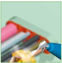
14) To smooth the surface of the NOFIRNO® sealant layer, a cloth is sprayed with water. This prevents the sealant from sticking to the cloth. Note: do not use soap water!
