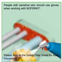
7) To smooth the surface of the NOFIRNO® sealant layer, a cloth is sprayed with water. This prevents the sealant from sticking to the cloth. Note: do not use soap water!
