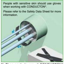
6) Then apply layers of CONDUCTON® flexible rubber strips 40 mm wide against the inside wall of the penetration. People with sensitive skin should use gloves when working with CONDUCTON®.
