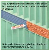
4) A 20 mm thick layer of NOFIRNO® sealant is applied on top of the ACTIFOAM®/ULTRA at the exposed side. Clean and dry the steel parts to apply the sealant on, and remove any dirt, rust or oil residues before applying the sealant.
